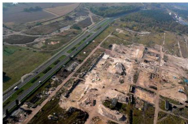
Fig. 2 Aerial view of “Polchem” after demolition ( http://archiwum.mpu-torun.pl/index.php?m=gal&id=13 )
